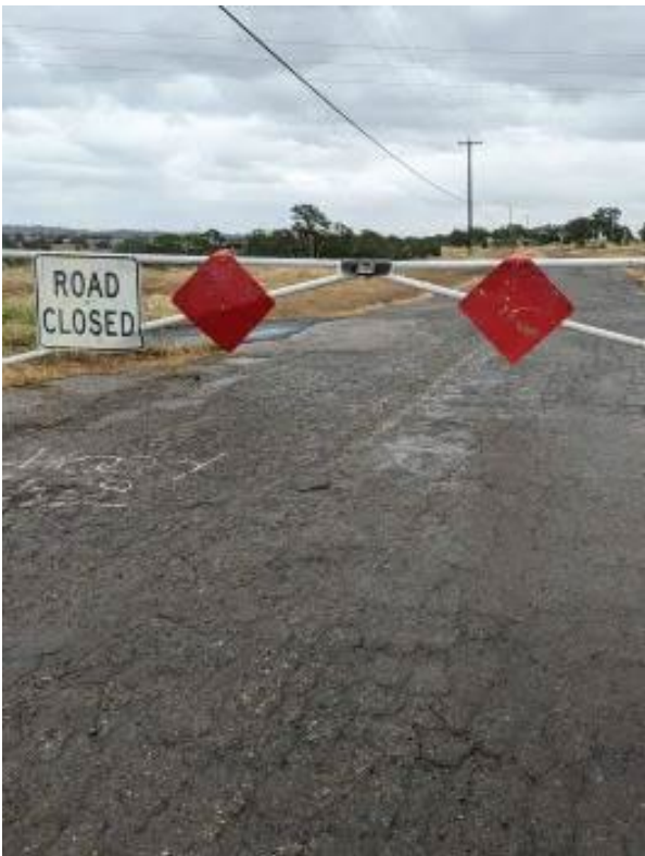
Upper Humboldt Rd Repaving
