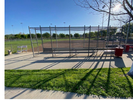
Back of dugout sections 3 rd base line- 5' x 6' (8 Sections)
